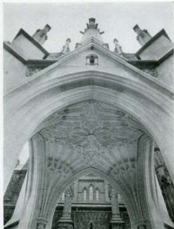
View Showing Groined Ceiling of Carved Buff Indiana Limestone in Soldiers' Memorial in Church Yard of St. James Church, Toronto, Ontario. Architects: Sproatt & Rolph.
