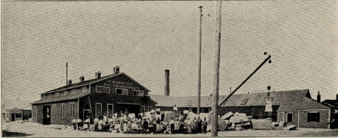
Exterior view of works.
