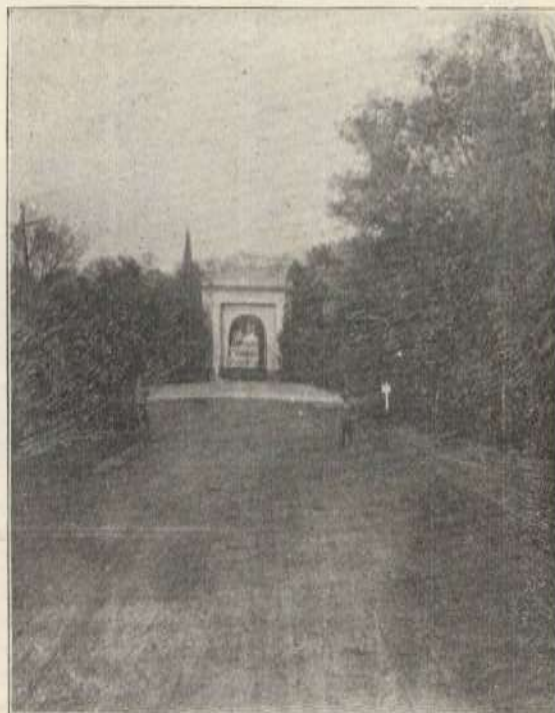
ENTRANCE, VICKSBURG NATIONAL CEMETERY.
