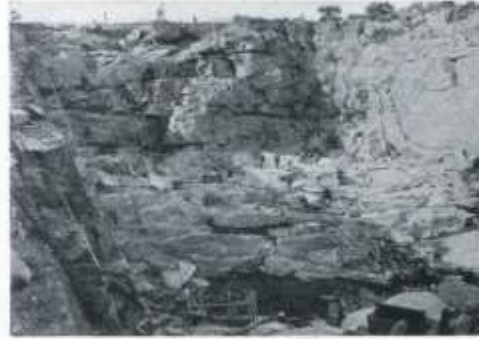
The Klondike Quarry Westerly
