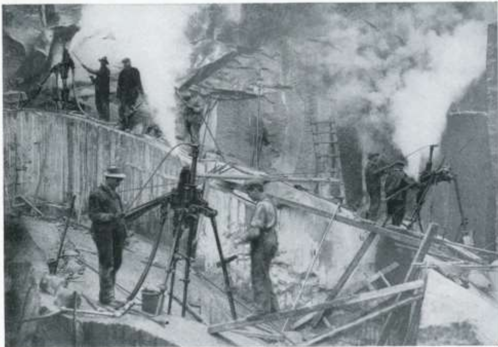
Sullivan Rock Drills and Quarry Bars at work; a close view. Note the cranking rods on the drills
