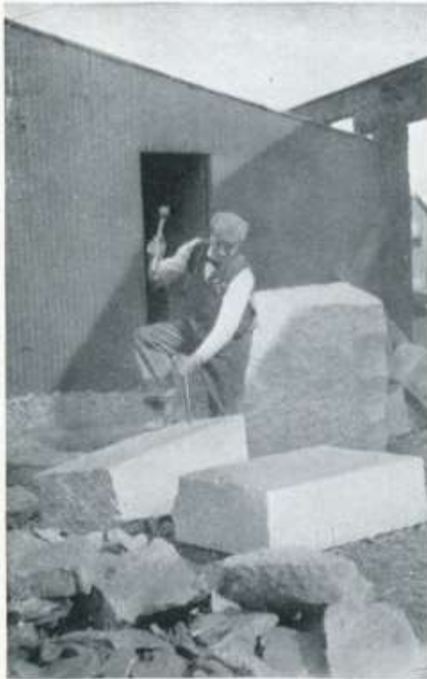
The old way of splitting granite at Westerly
