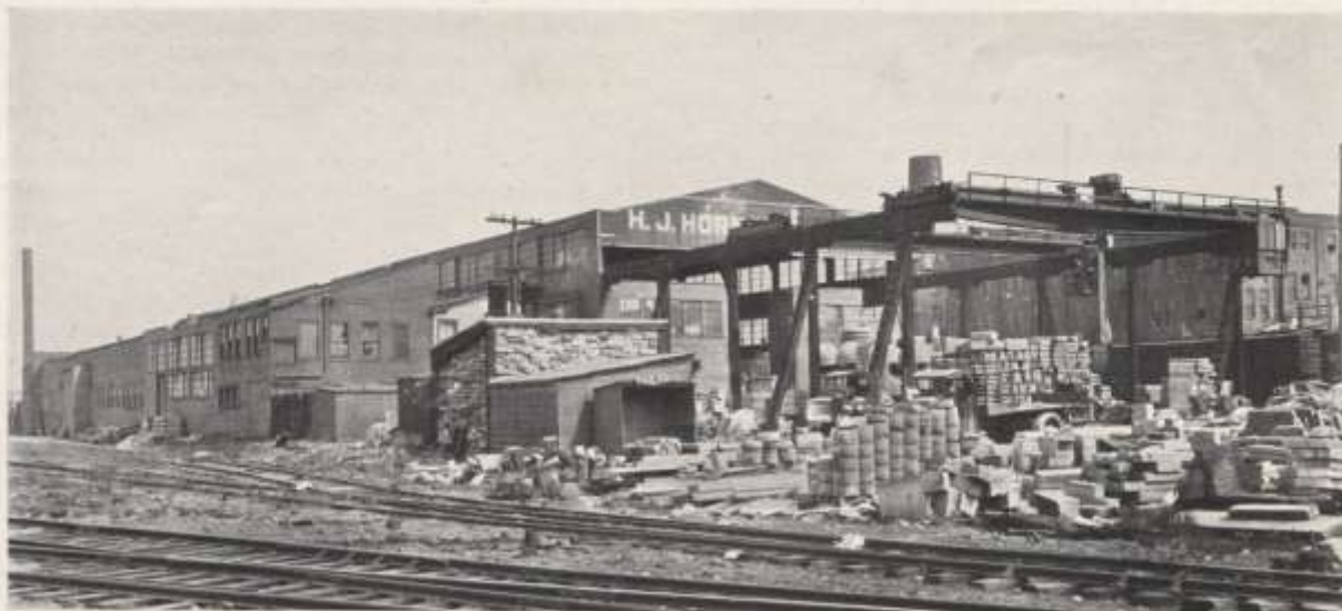
Cut Stone plant of H. J. Horner & Sons, Lister Avenue, Newark, N. J.
