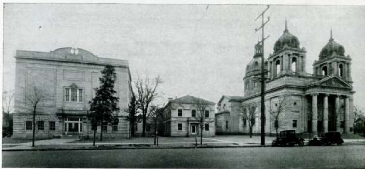
St. Mary's Cathedral Group, Wichita, Kansas, consisting of the Cathedral, High School, Gymnasium and Rectory, Constructed in Buff Indiana Limestone. Architects: Masqueray and Schmidt, Boucher & Overend.
