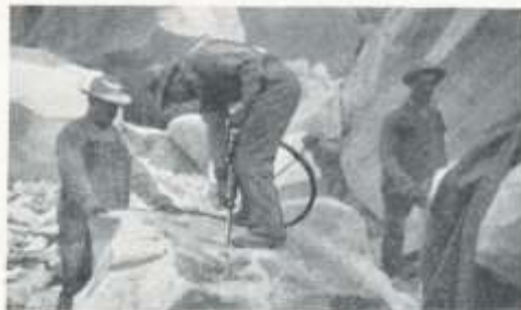
Splitting stone for paving blocks in an Ohio quarry
