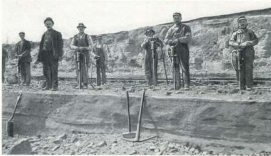
Sullivan "DB-19" hammer drills on a shallow bench, Shenango Limestone Co.
