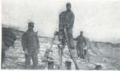
Sullivan rock drill on bench, Shenango Limestone Co.
