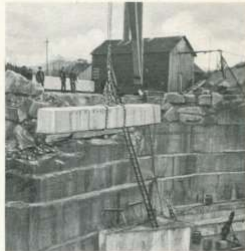
Hoisting a 40-ton block of marble from the South Dover quarry.
