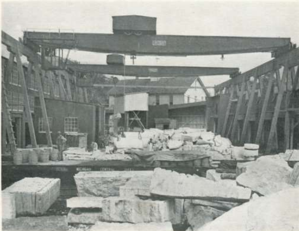
The craneway and finishing works, South Dover Marble Co.
