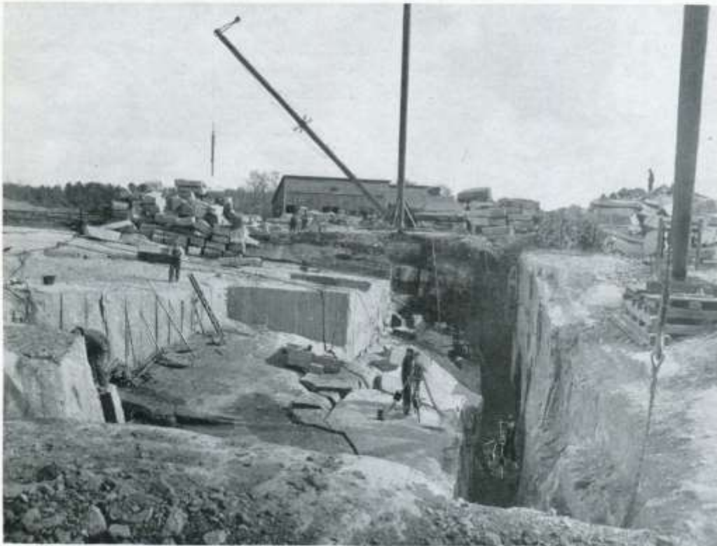
Quarry No. 3, Sauk Rapids Granite Company. Sullivan Tripod Drills at work
