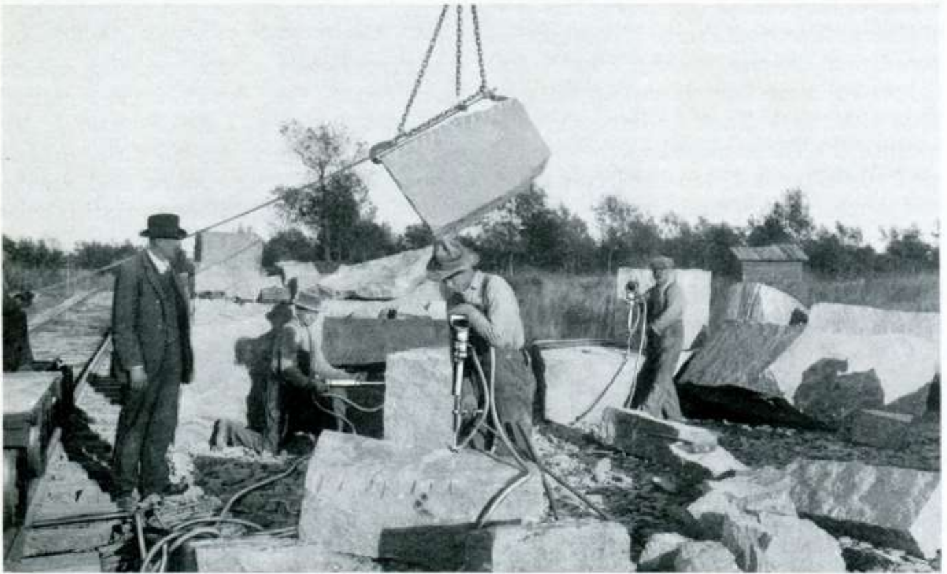
Sullivan Plug Drills at work, Sauk Rapids Granite Company
