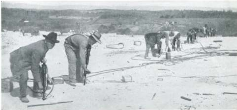
Starting a 400-foot ledge line with Sullivan Plug Drills
