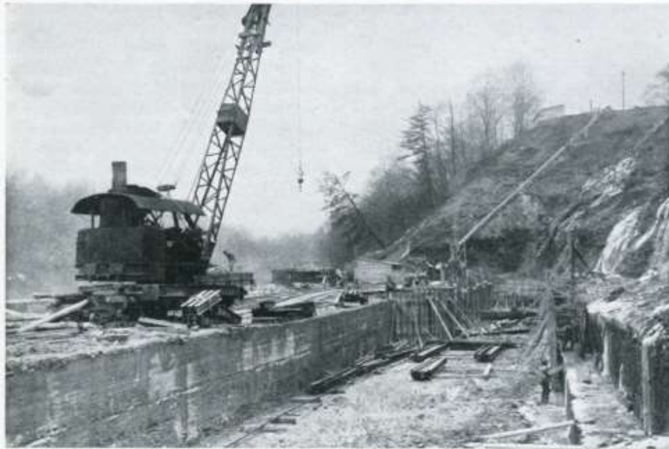
Ash pit, Northern Ohio Power Co. Channeled wall at left
