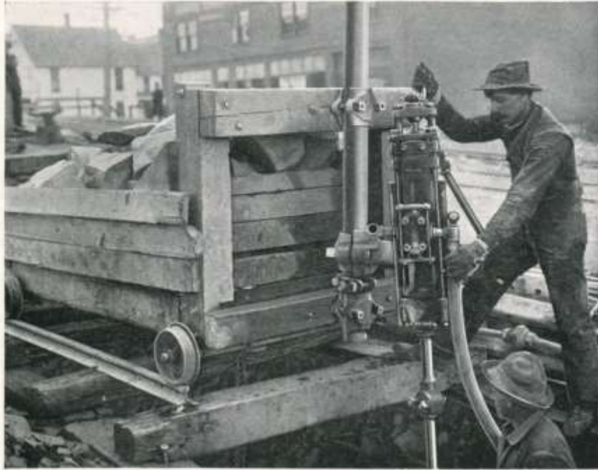
Sullivan Drill and home made trench drilling rig
