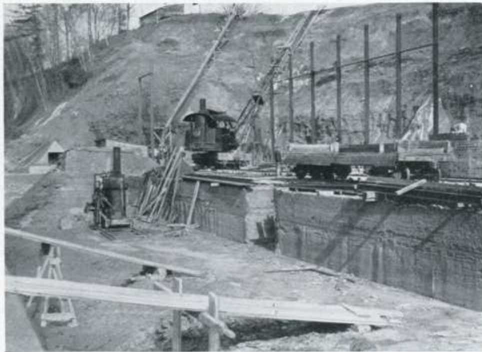
Beginning the condenser well. First bench. Sullivan Channeler at left
