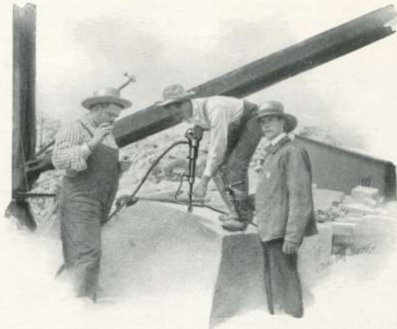
Sullivan "Plug Drill" on a test run.
