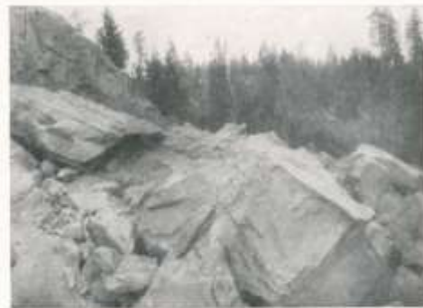
Hercules Quarry after a blast
