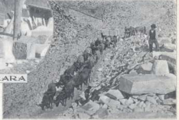
HOW THE QUARRIED MARBLE IS CARRIED DOWN.
