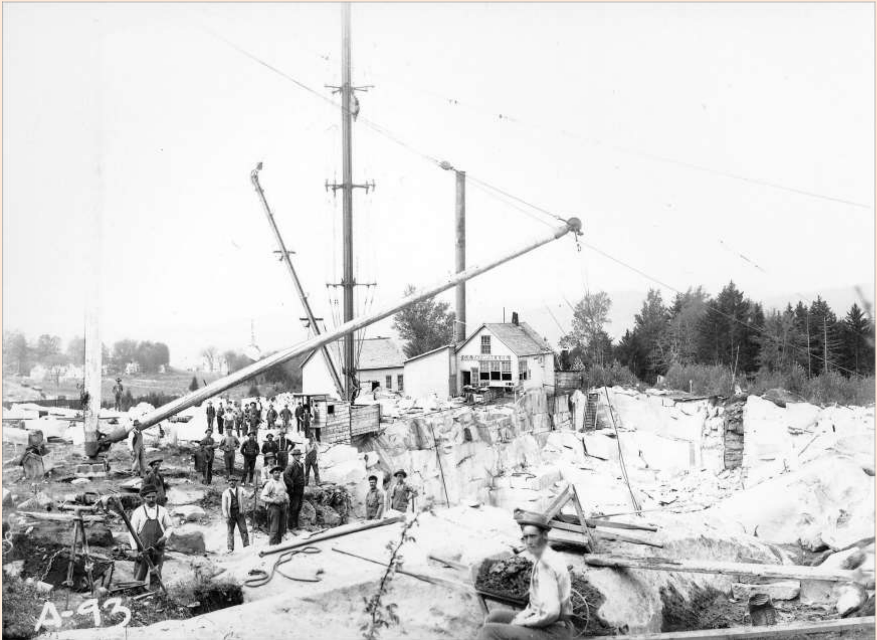
“This circa 1895 photo of the C.E. Tayntor quarry shows the largest derrick in the world in the center.” (Photo from the collection of Todd Paton.)
