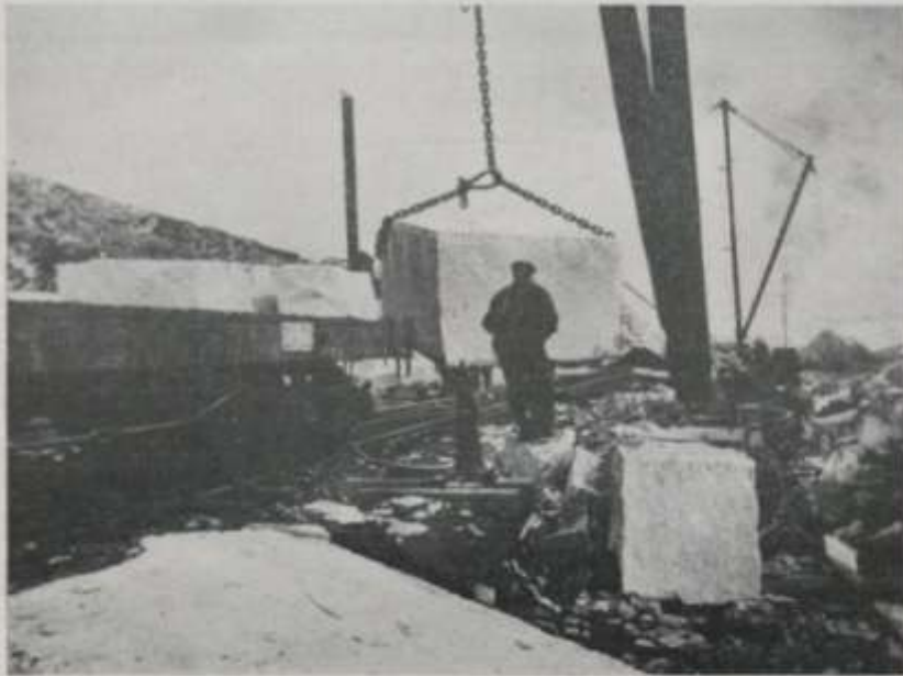
View on the bank at the Barclay quarries, showing a nice pattern being loaded.
