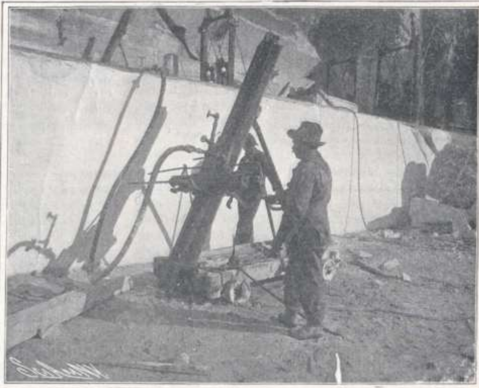
Type of Steam Drill Used in Quarrying.
