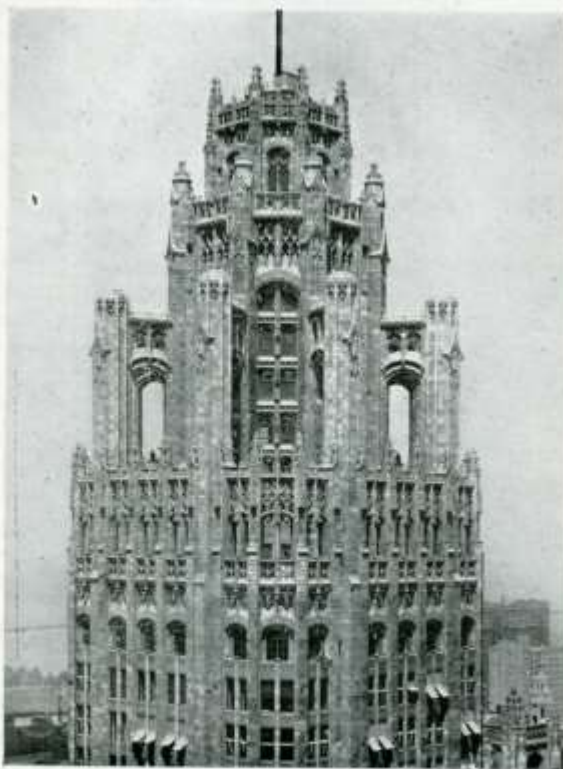
Tower of the Chicago Tribune Building, showing Beautiful Effects of Carved and Ornamented "Old Gothic" Indiana Limestone. J. Hoadley & Sons Co., Cut Stone Contractors. Howell & Hood, Architects.
