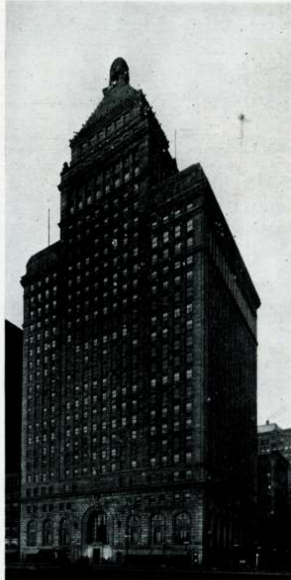
S. W. Straus Building, Chicago, as Seen from Grant Park. Architects: Graham, Anderson, Probst & White. Exterior of Select Buff and Variegated Indiana Limestone furnished by the Indiana Quarries Company. Cut Stone Contractors: The Central Oolitic Stone Company.
