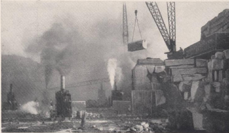
The Hoosier Quarry on a busy day; Sullivan Duplex Channeler in foreground
