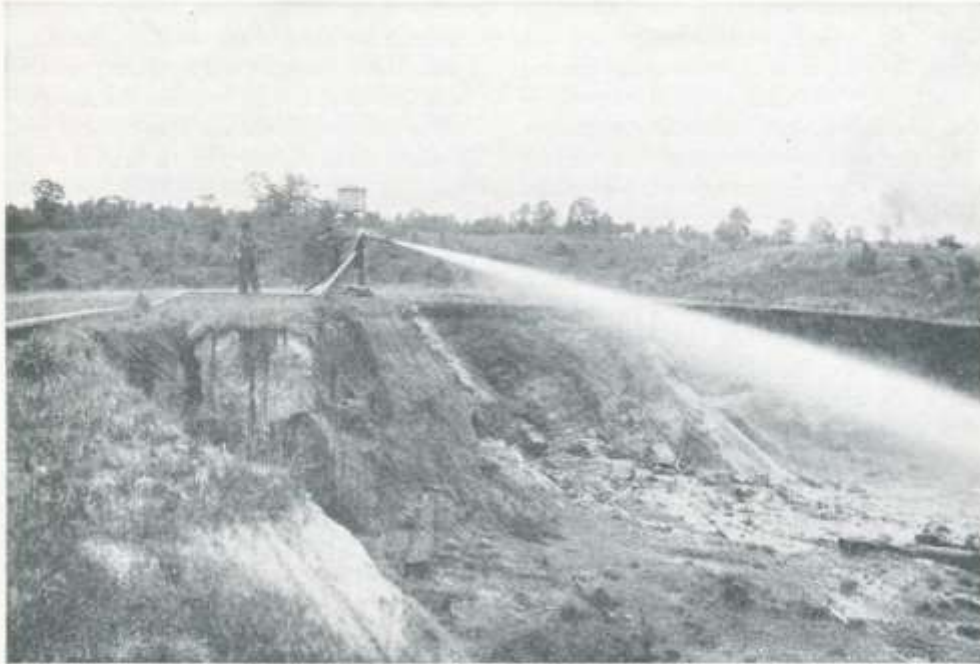
A hydraulic stripper at work.
