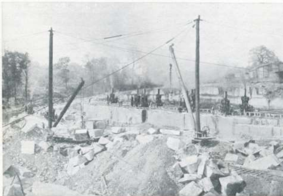
Ten Sullivan channelers in a well developed quarry.
