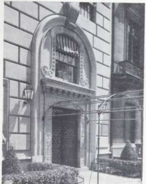
Ornate Entrance of Apartments at 956 Fifth Avenue at 77th Street. The Material Is Indiana Limestone. Architect: Nathan Korn.
