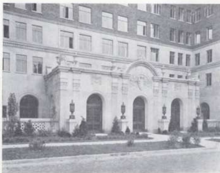
Entrance Detail of the New Belvedere Apartments, Cincinnati, in Which Indiana Limestone Was Used Exclusively. Architect: C. H. Ferber.
