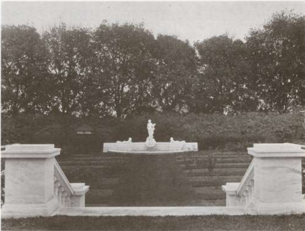
Sunken Garden on an estate at Fairfield, Connecticut. Mountain White Danby marble, from Vermont, was used.
