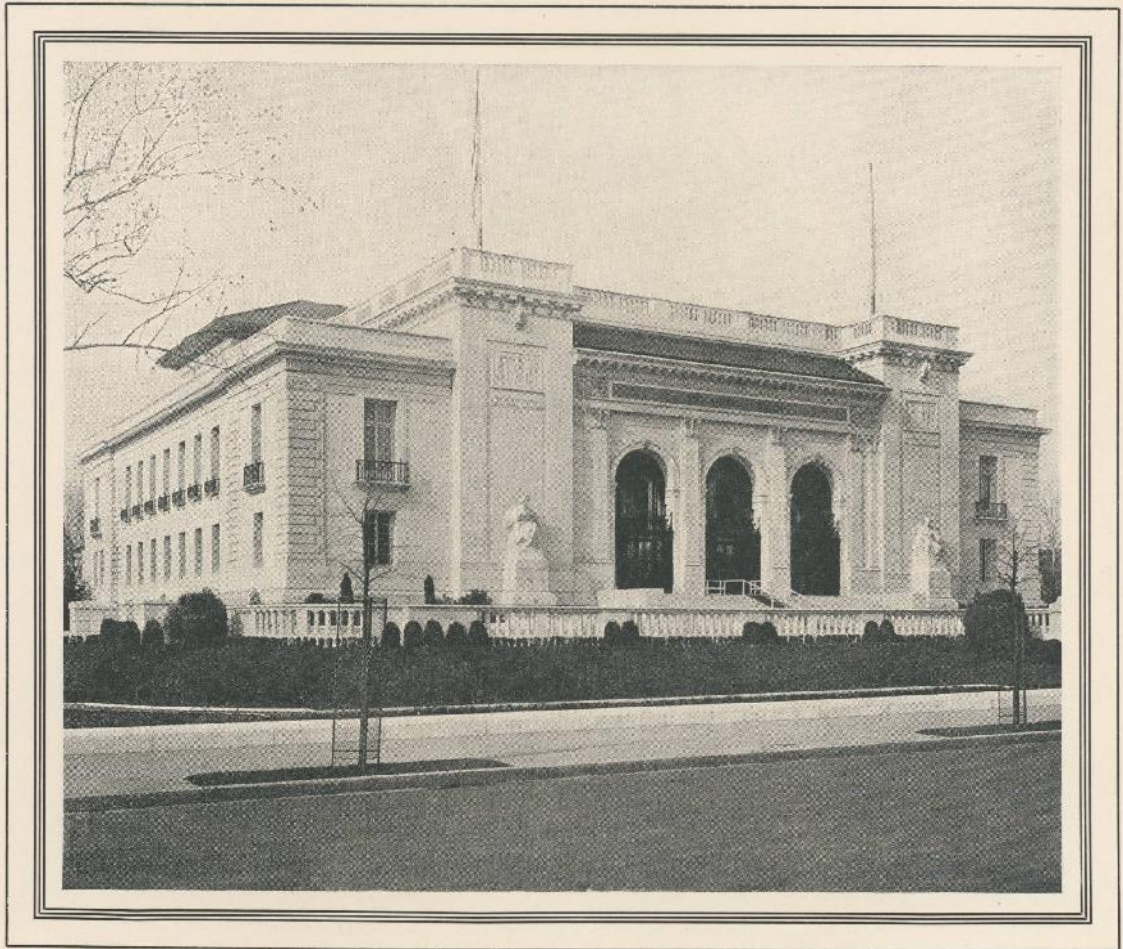
PAN AMERICAN BUILDING, WASHINGTON, D. C., THE INTERNATIONAL CAPITOL. ENTIRE BUILDING, INCLUDING SCULPTURED FIGURES, OF GEORGIA MARBLE. THE DESIGN SELECTED AFTER AN ARCHITECTURAL COMPETITION, WAS PRODUCED BY ALBERT KELSEY AND PAUL P. CRET. GROUPS ON EITHER SIDE OF THE MAIN ENTRANCE BY CUTZON BORCLUM AND ISIDORE KONTI.
