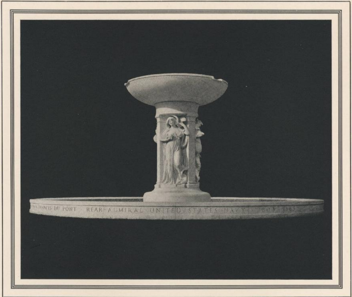
DU PONT MEMORIAL FOUNTAIN, WASHINGTON, D. C., ERECTED TO COMMEMORATE THE SERVICES OF ADMIRAL DU PONT. THE PEDESTAL IS CUT FROM A SINGLE BLOCK OF GEORGIA MARBLE 10 FEET HIGH. THE BOWL REQUIRED A BLOCK OF GEORGIA MARBLE 13 FEET IN DIAMETER. HENRY BACON, ARCHITECT. DANIEL CHESTER FRENCH, SCULPTOR. CARVING AND ERECTION BY PICCIRILLI BROS.
