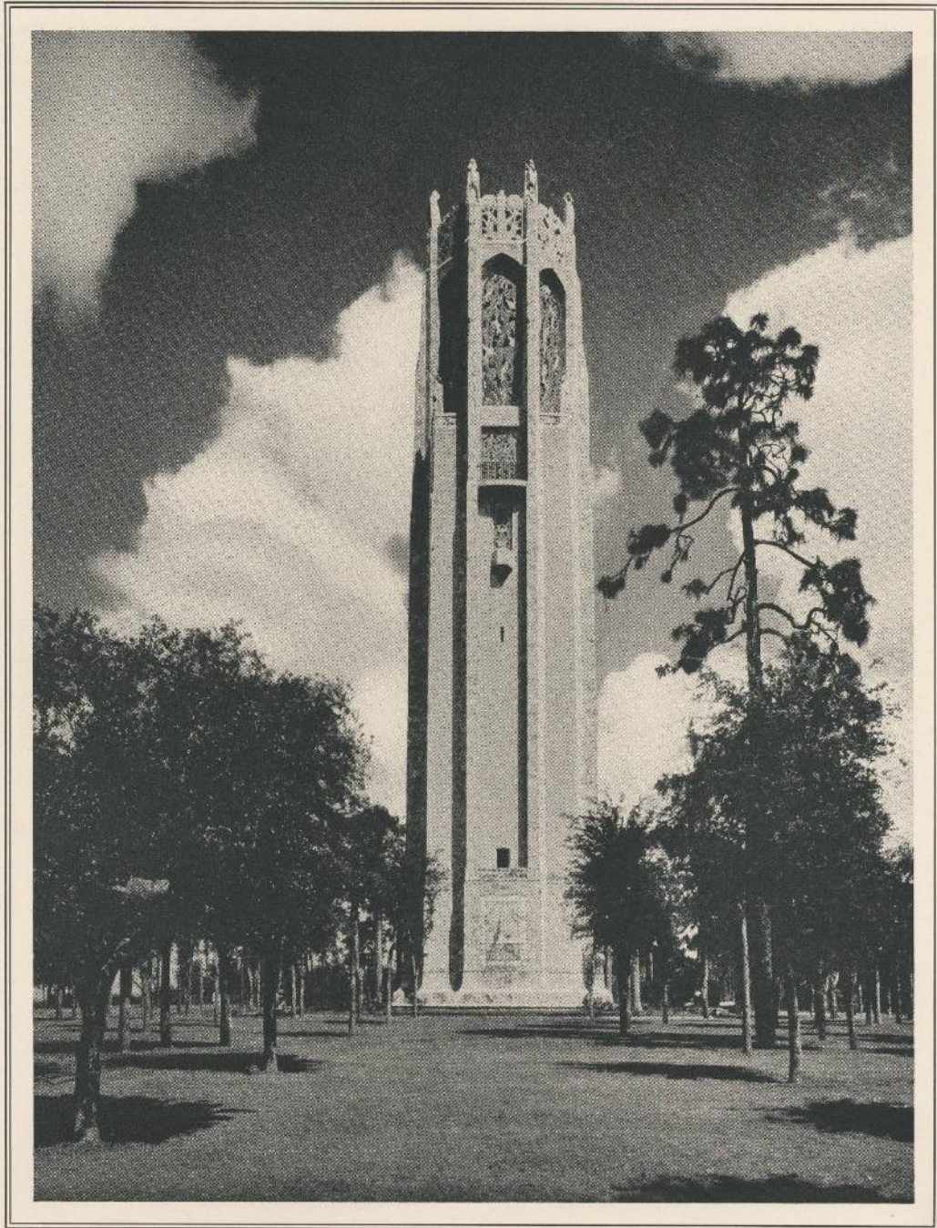
THE BOK CARILLON, OR "SINGING TOWER," AT MOUNTAIN LAKE, FLORIDA, CON- STRUCTED OF PINK AND CREOLE GEORGIA MARBLE, AND TAN COQUINA ROCK. THE CARVED HERONS ON THE PEDIMENT OF THIS STRUCTURE ARE 14 FEET HIGH, AND ARE CARVED FROM SOLID BLOCKS OF PINK GEORGIA MARBLE. MILTON B. MEDARY, ARCHITECT, AND LEE LAWRIE, SCULPTOR.
