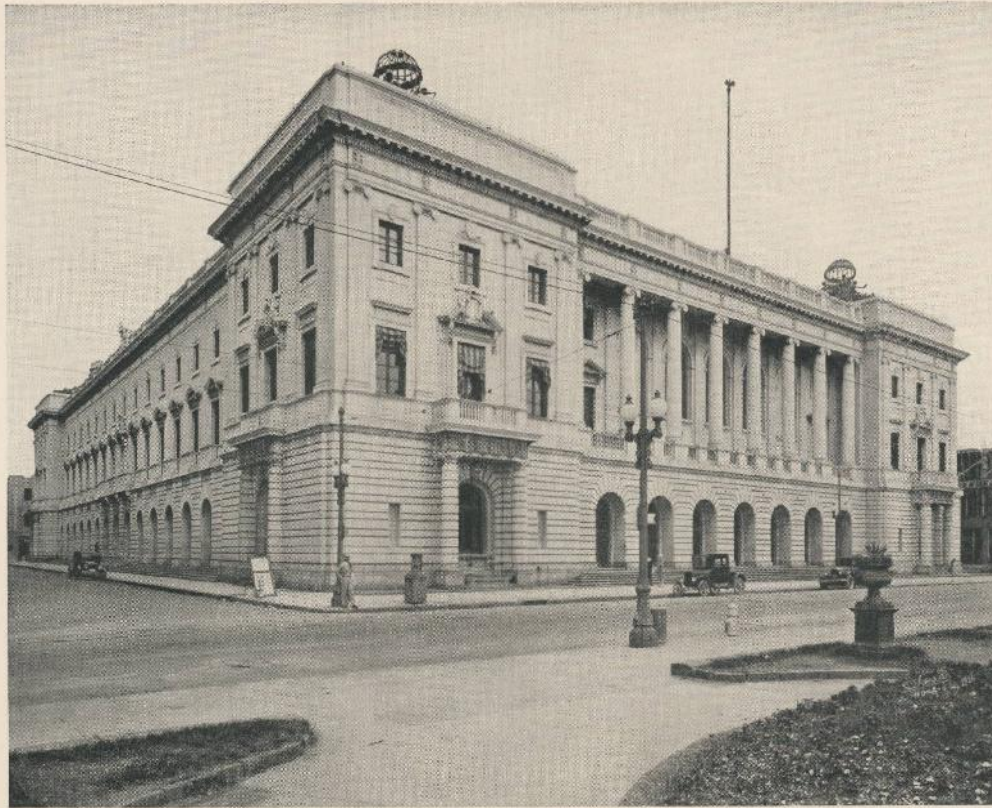
FEDERAL BUILDINGS ARE IN A GREAT NUMBER OF INSTANCES CONSTRUCTED OF GEORGIA MARBLE. GEORGIA MARBLE IS THE ONLY MARBLE WHICH THE FEDERAL GOVERNMENT DOES NOT REQUIRE TO BE WATERPROOFED WHEN USED FOR EXTERIORS. ABOVE—POST OFFICE, NEW ORLEANS, LOUISIANA. JAMES GAMBLE ROGERS, ARCHITECT.
