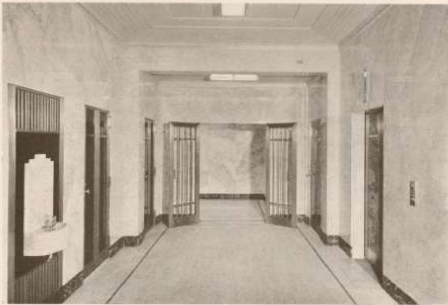
For the first floor elevator lobby, Pittsburgh Federal Reserve Bank, the walls are of Silver Gray Siena, with Marion Gray base. The floor field is Roman Travertine.
