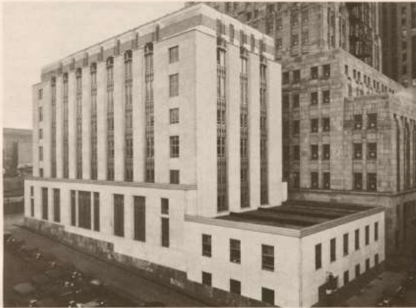
Upon a base of Dark Creole Georgia marble, the walls of Light Cherokee Georgia marble rise to the uniquely designed attic story.
