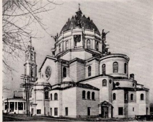
Rear of National Shrine of Our Lady of Victory's Care, showing massive proportions of structure and height of dome and twin towers rising 185 feet above level. Exterior entirely of White Georgia Marble furnished by the Georgia Marble Company. Architect: Emile M. Ulrich.
