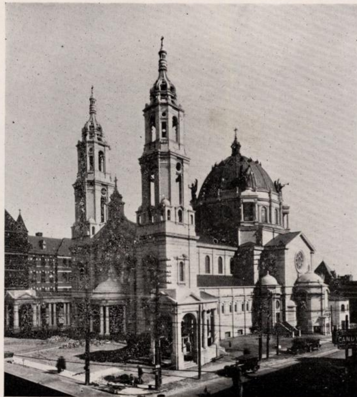
New Church of The National Shrine of Our Lady of Victory's Care, Lackawanna, N. Y. Exterior of White Georgia Marble furnished by the Georgia Marble Company. Architect: Emile M. Ulrich, Cleveland, Ohio.
