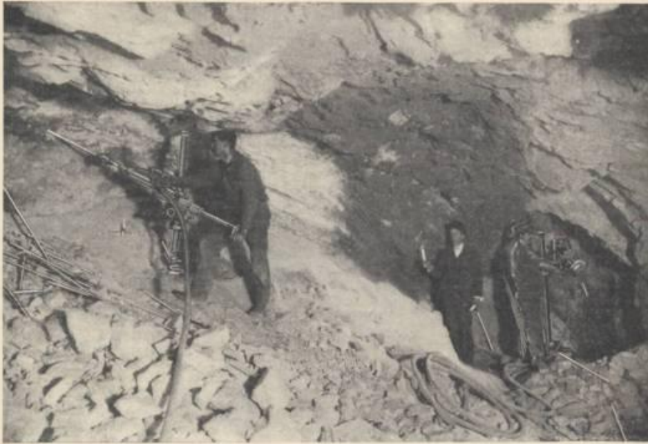
Sullivan "U S" rock drills in an Arizona stope.
