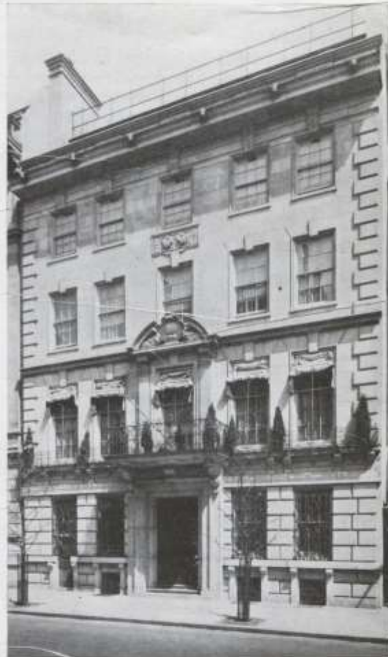
RESIDENCE OF JOHN T. PRATT, NEW YORK At 9 and 11 East Sixty-first Street. Architect: Charles A. Platt, New York. Cut stone contractors: George Brown & Co., Newark. Built of Buff Indiana limestone
