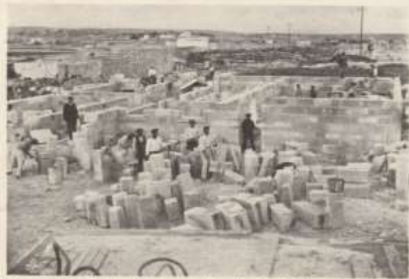
Erecting a Small House on Island of Malta, showing construction methods with walls rising from the ground level. All of the work is done by hand.
