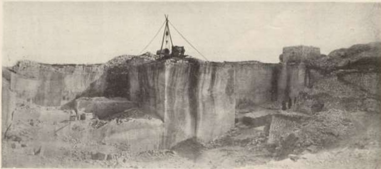
The Tad-Daul Limestone Quarry on The Island of Malta, from which about 1,500,000 cubic feet of blocks were taken in 1918-21 for construction of Mediterranean Seaplane Base and barracks at Calafra, Malta. All of this stone was quarried by hand. This and other photographs used through the courtesy of C. Darmanin & Son.
