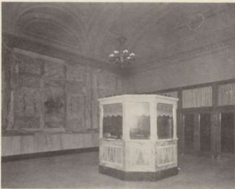
Vestibule of new Missouri Theater, St. Louis, showing Wainscoat of Eastman's Cipoline; Base of Imported Verde Antique, and booth of Alabama Madre Veined Marble. Pickel Marble & Granite Co., marble Contractors. Marble furnished by the Tompkins-Kiel Marble Co.
