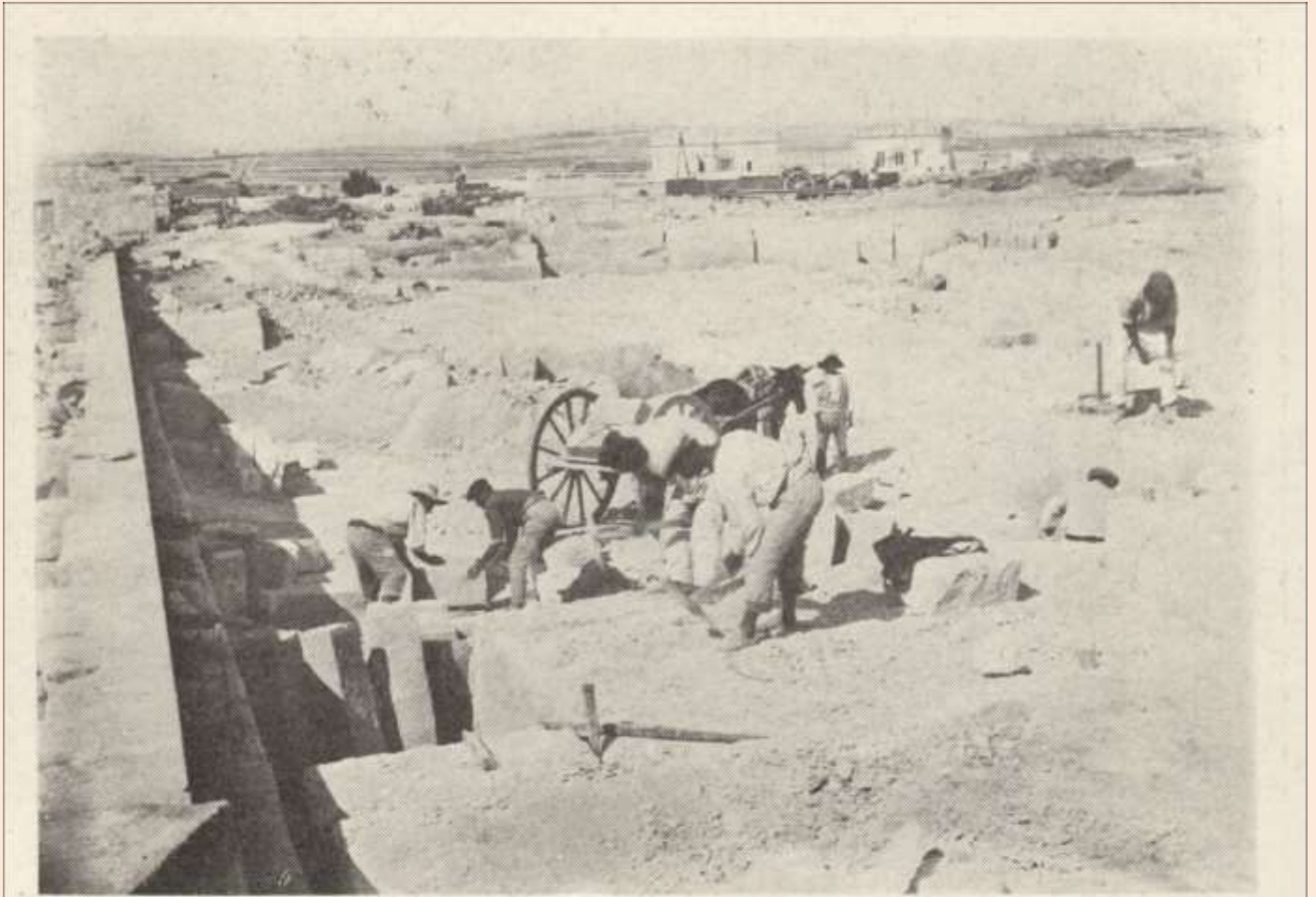
Opening a new Quarry of Malta Limestone, Island of Malta. Wedges are used to loosen the blocks. No machinery is used.
