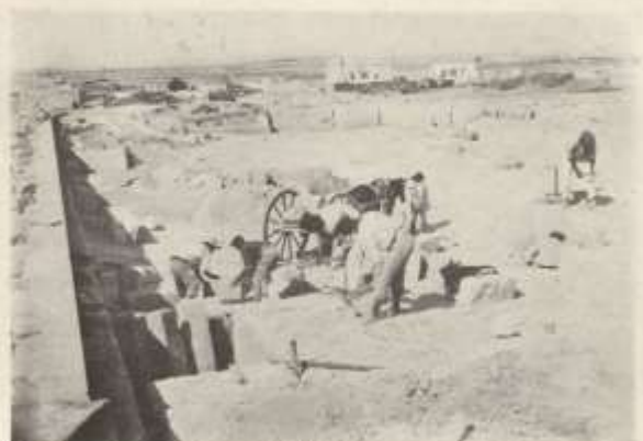
Opening a new Quarry of Malta Limestone, Island of Malta. Wedges are used to loosen the blocks. No machinery is used.
