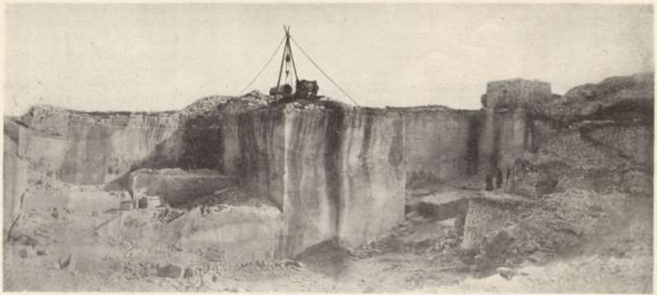
The Tad-Daul Limestone Quarry on The Island of Malta, from which about 1,500,000 cubic feet of blocks were taken in 1918-21 for construction of Mediterranean Seaplane Base and barracks at Calafrana, Malta. All of this stone was quarried by hand. This and other photographs used through the courtesy of C. Darmanin & Son.
