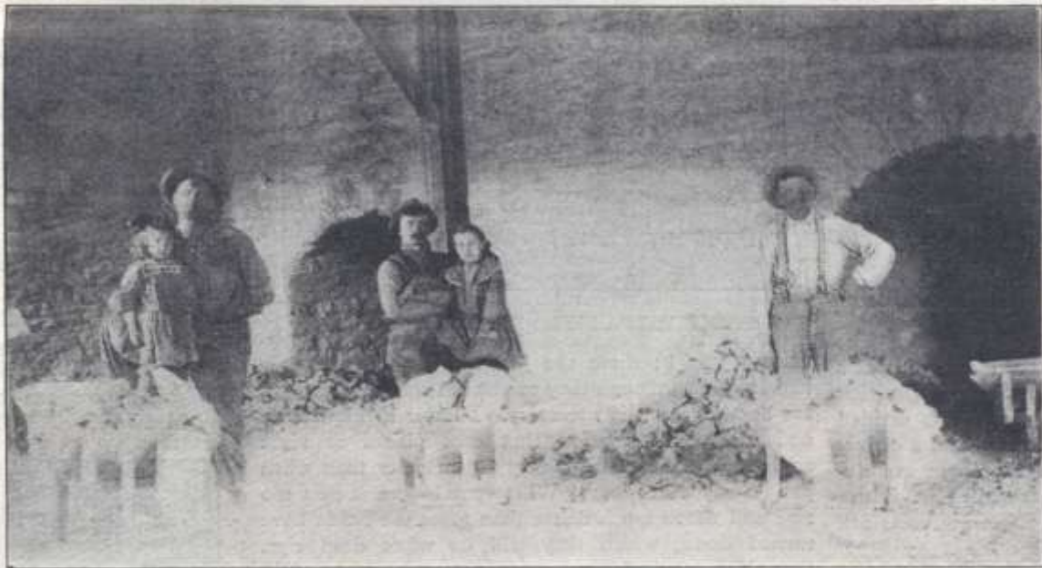
DRAWING OFF THE LIME FROM THE KILNS. FIG. 263.
