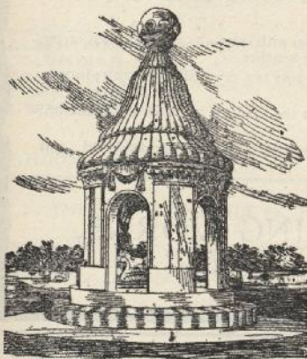
Blocher Mausoleum, erected by McDonnell & Sons.
