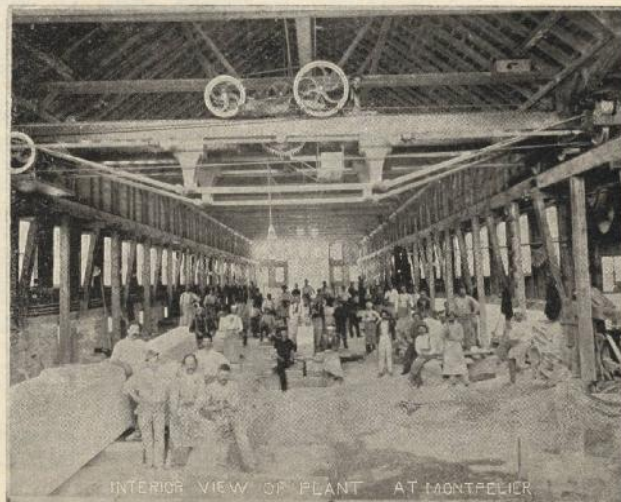
INTERIOR VIEW OF PLANT AT MONTPELIER.
