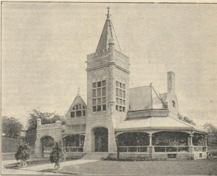
SUPERINTENDENT'S OFFICE AND WAITING ROOMS, CAVE HILL CEMETERY.
