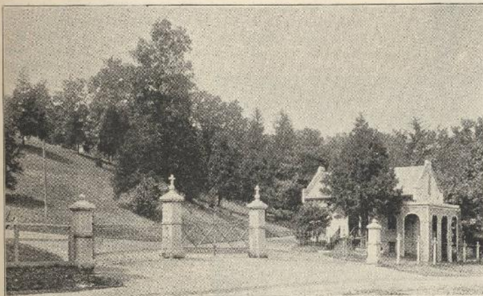
ENTRANCE AT BROADWAY.
