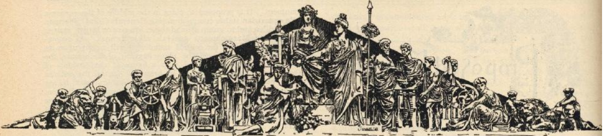
PEDIMENT ON MACHINERY HALL, WORLD'S FAIR —PEABODY &amp; STEARNS, ARCHITECTS.
