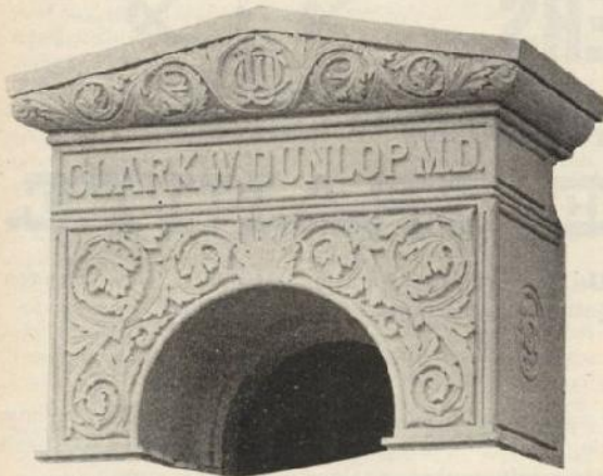
Portion of entrance to Vault in Woodlawn Cemetery, N. Y.
