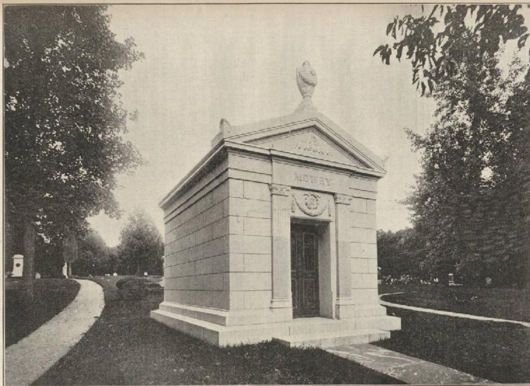
The above is a cut of a Vault erected last spring in Englewood, N. J. Stock is fine grained mediam Barre, cut and finished with Pneumatic Stone Dressers, by Chas. H. More & Company at their Montpelier plant. While plain and simple in its outline, it is in good proportion and well constructed. The outer surface being all hammered, presents a smooth and unbroken surface to the weather, thus preventing any lodgment of dust and other matter to mar or discolor its beauty. On this account, plain hammered work is far superior to rock face or rustic work, either in Monuments or Mausoleums of this kind. For sizes and prices, please apply to CHAS. H. MORE & CO., Barre, Vt. , or to their Chicago office at 53 Dearborn St.
