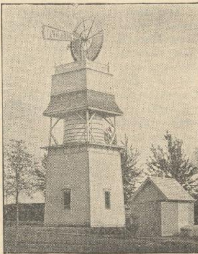
WIND MILL AND TANK.
