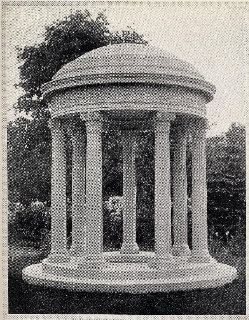
Work of Joseph Newall & Co., New York City. Cut by Joseph Coduri Granite Company Westerly, Rhode Island
