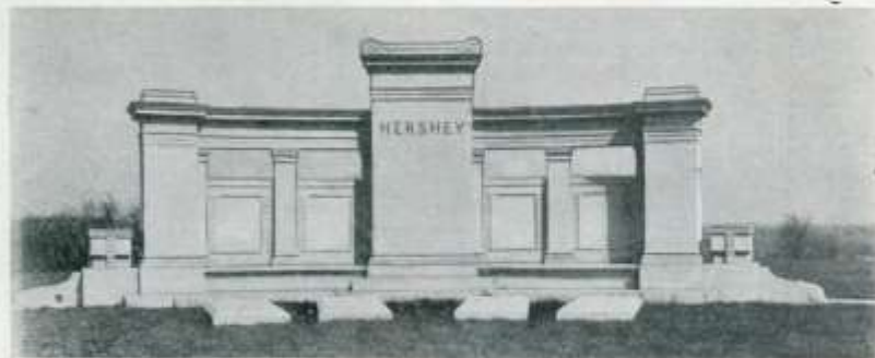
MASSIVE EXEDRA SCREEN OF IMPRESSIVE LINES. Haldy Marble and Granite Wks., Lancaster, Pa., Contrs.
