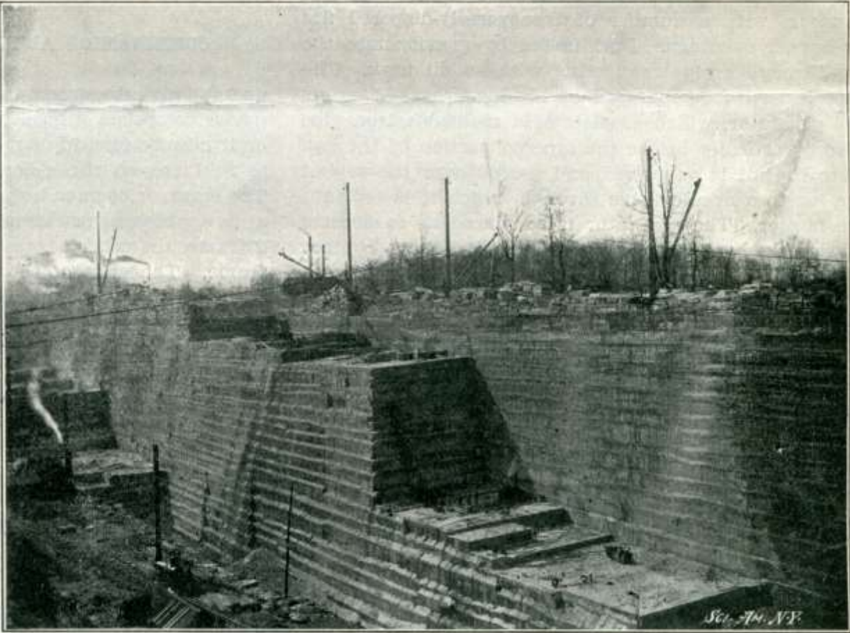
Sandstone Layers in an Ohio Quarry.
