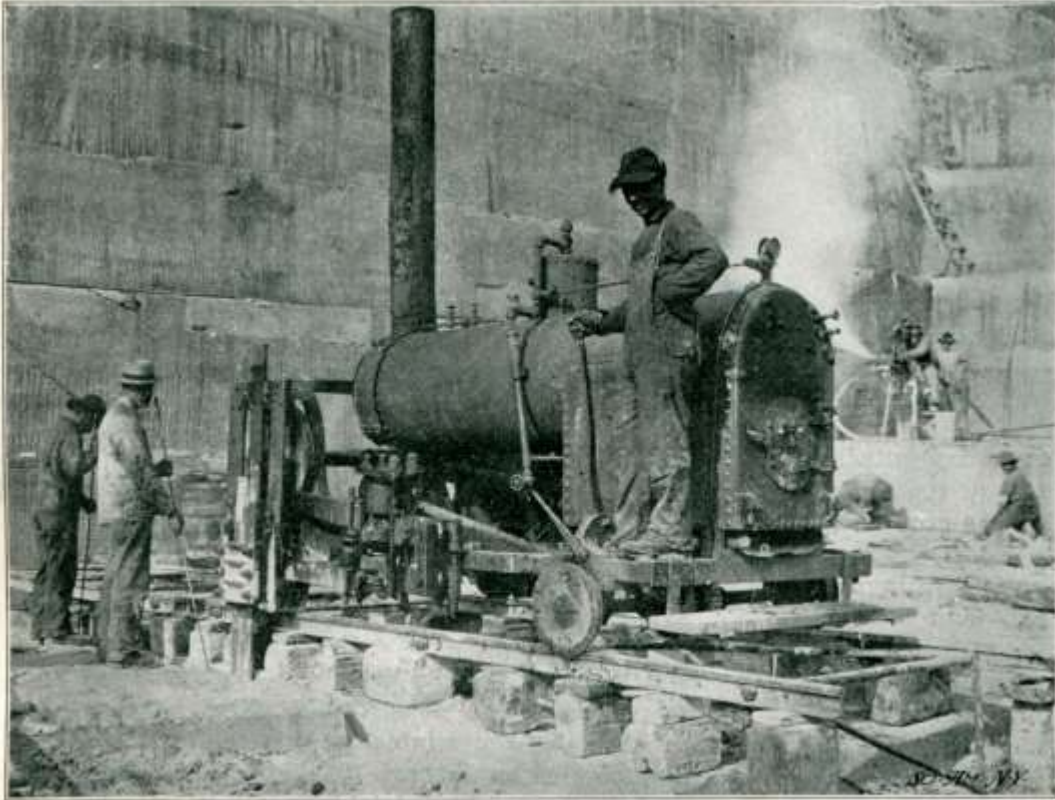
Sawing Sandstone by Machinery.
