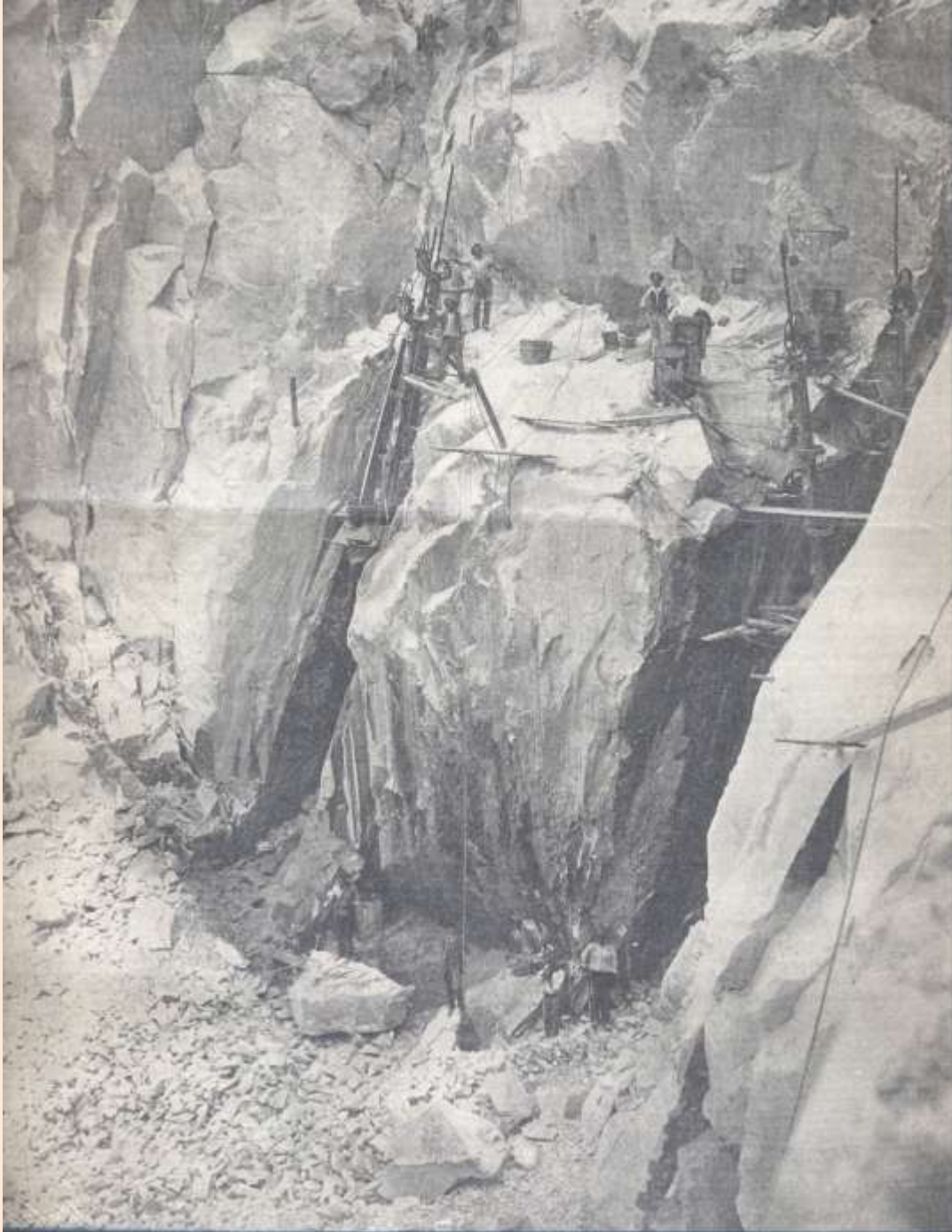
“Miners Making the Electrical Connections for Blasting a Monster Block of Carrara Marble”
