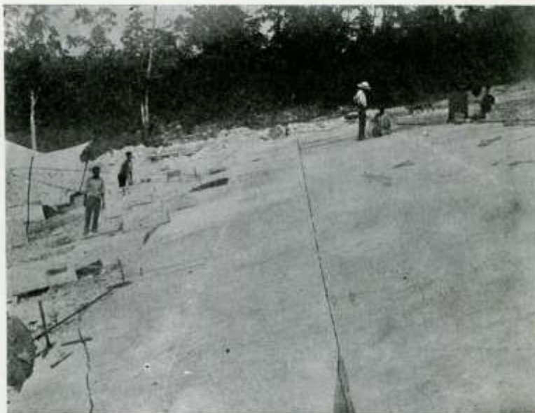
A "LIFT" BEING SPLIT AND DRILLED INTO REQUIRED WIDTHS AND LENGTHS.
