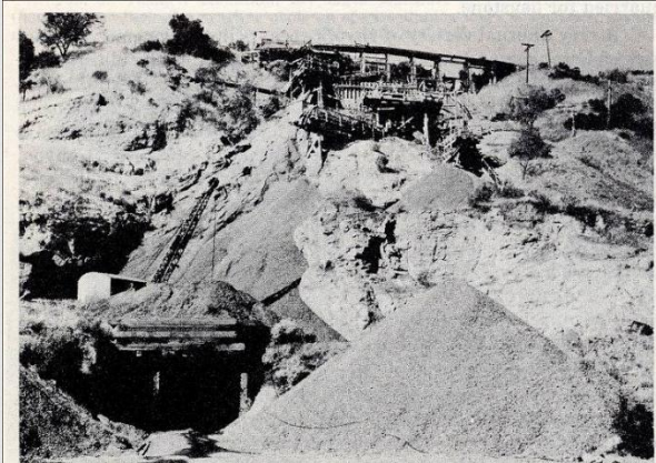
FIG. 12. J. M. Nelson quarry, near Cordelia, Solano County. General view of crushing and screening plant and stock pile of crushed basalt.
