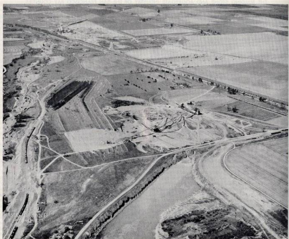
FIG. 1. Pacific Coast Aggregates Company operation near Livermore, Alameda County. Rock, sand, and gravel are scraped from surface deposits by heavy earth-moving equipment, each unit carrying 20 tons. Material is gathered in a sub-surface hopper, fed onto a conveyor belt, and run through a washing, screening, and crushing plant. Sized material is then sent to stock piles via conveyor belts. Belt conveyors also connect the rail and truck-loading hoppers with the stock piles. In the background is the gravel pit and plant of Henry J. Kaiser Company. Photo by Clyde Sunderland, Oakland.
