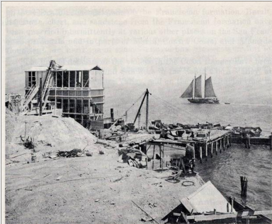
FIG. 2. An old photograph of the Healy-Tibbets rock quarry crushing plant and loading dock near Winehaven, west of Richmond, Contra Costa County. Crushed rock once was shipped by barge in large open boxes as shown in the left middle ground. Quarry was in sandstone of the Franciscan formation. Site is now occupied by installations connected with the Standard Oil Company refinery at Richmond. Photo courtesy Pacific Gas and Electric Company.
