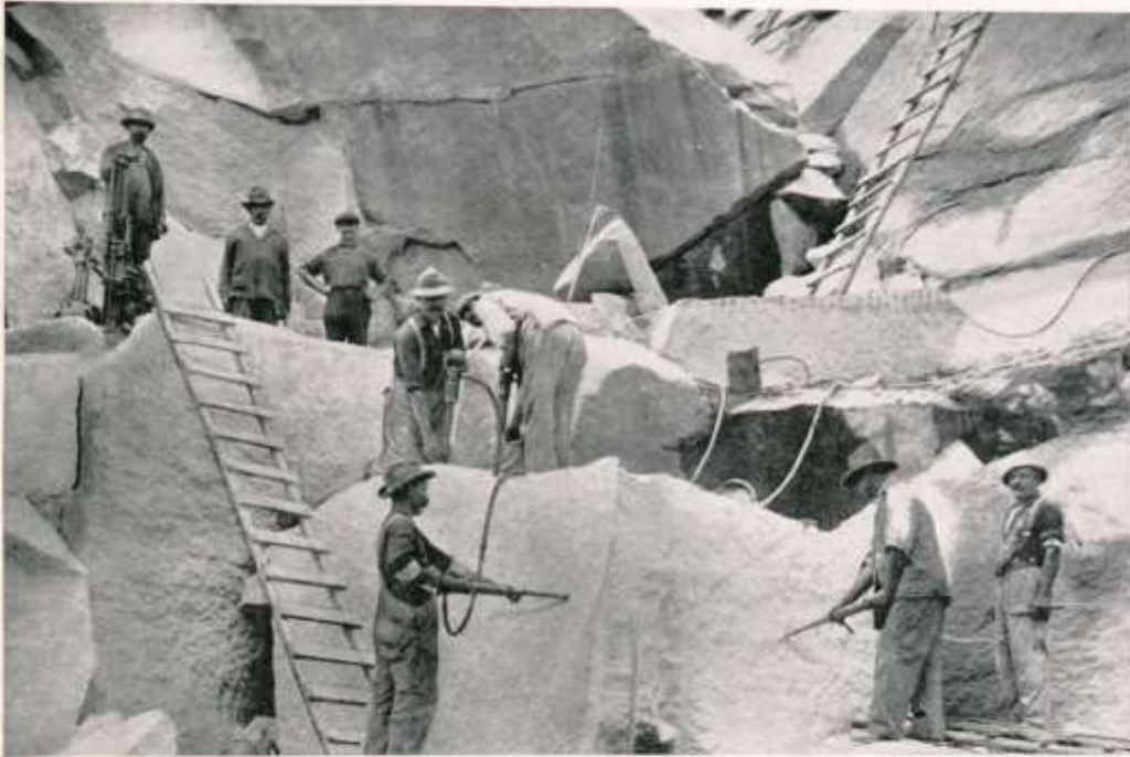
Splitting granite at Milford with Sullivan Plug Drills, for the Perry Memorial
