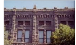
Upper story of the Digg's building in Woodland built of Ventura Co. Sandstone
