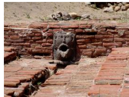
Gargoyle Waterspout in the Mission San Luis Rey de Francia Lavandería, photo by Nicole McClellan
